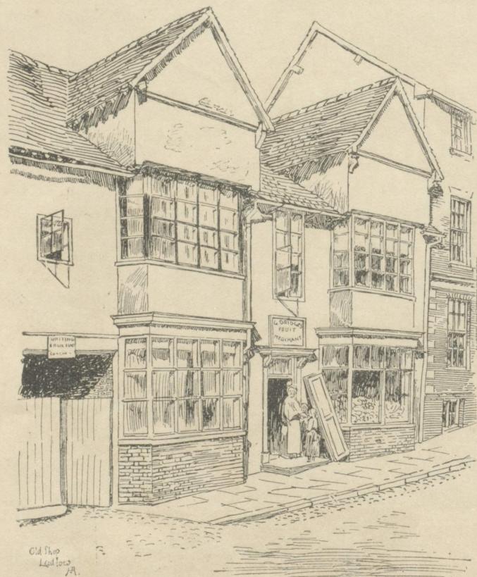
EARLY EXAMPLE OF THE USE OF GLAZING BARS, LUDLOW.
