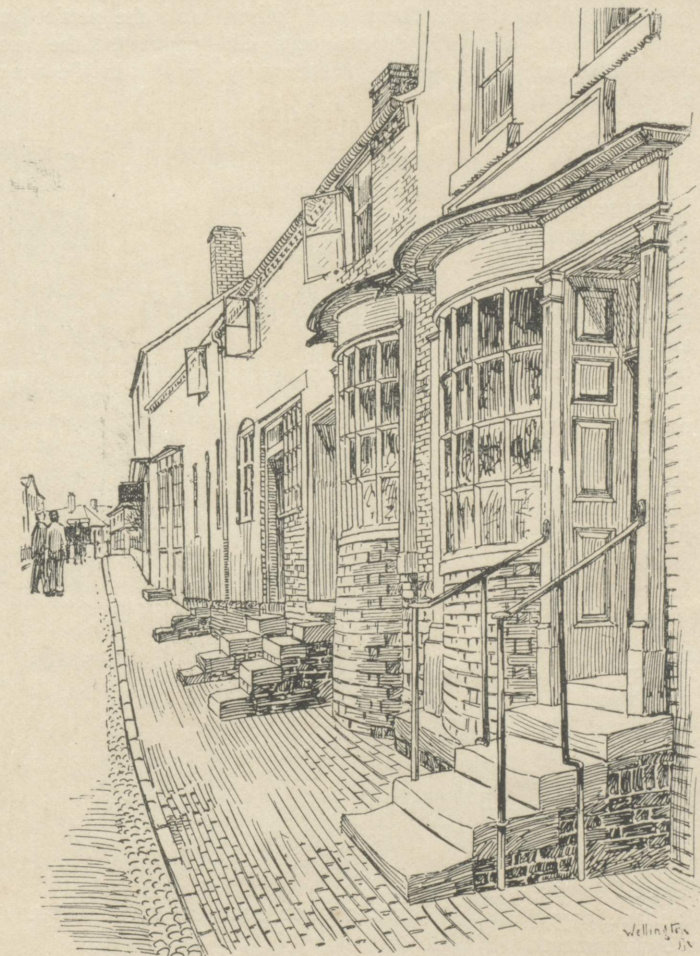
SHOP FRONTS AT WELLINGTON, SALOP, EIGHTEENTH CENTURY.
